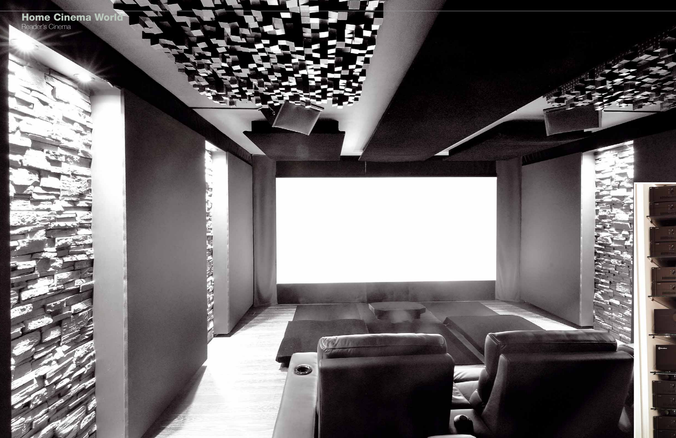
The ceiling is acoustically optimized with meter-long absorbers and so-called „Skyliners,“ which act as diffusers
