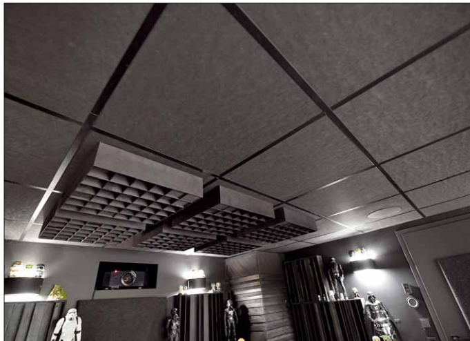
The acoustic ceiling is suspended by around 30 centimeters. Six diffusers are placed on it to provide more „room height“ above the seats.
